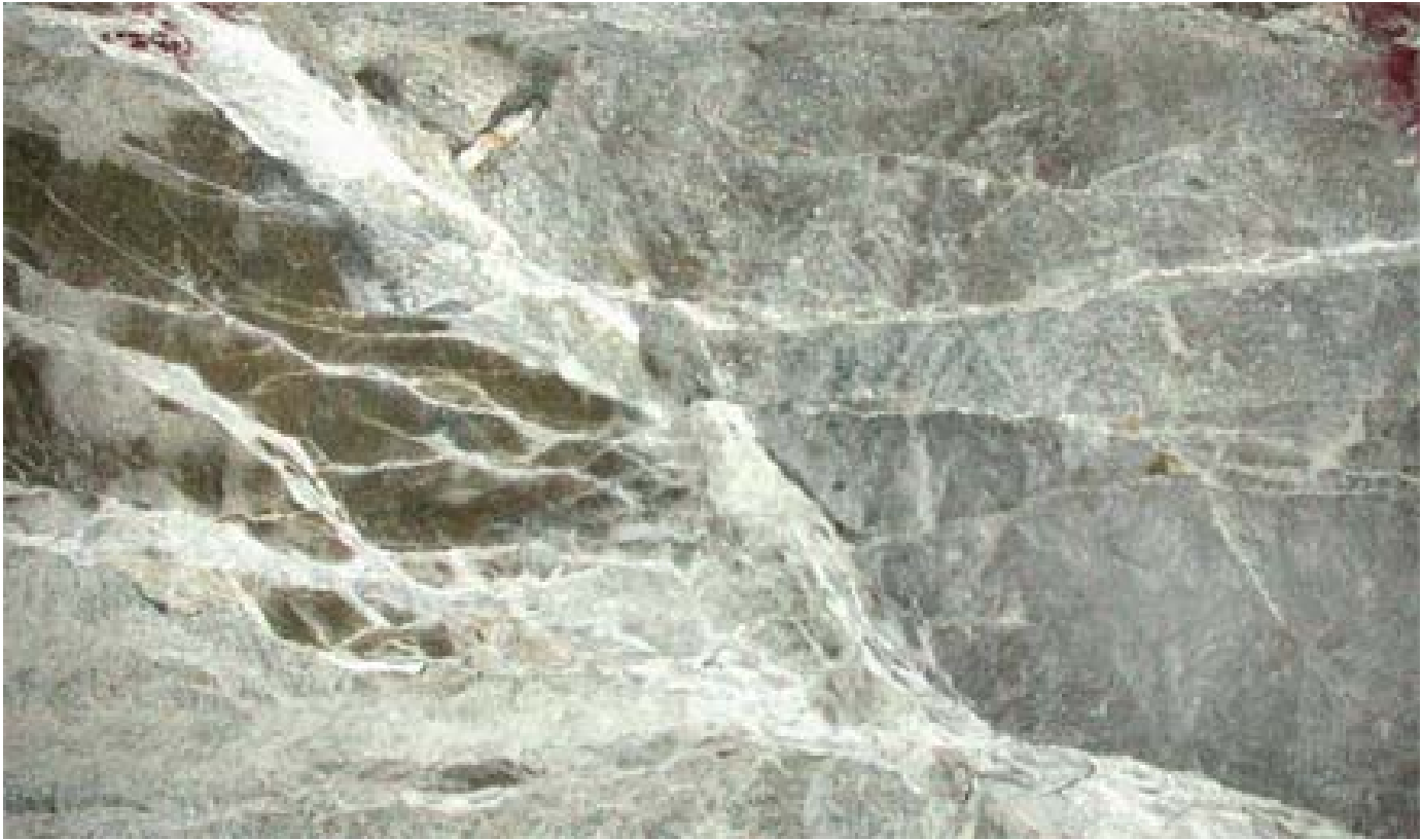
Fig. 7. View on tunnel's roof in the Bosman fault-zone. Note dense pattern of cross-cutting, zigzagging slip-surfaces of several scales; width of photo is about 1 m (see also figures in [3] and [5]).
