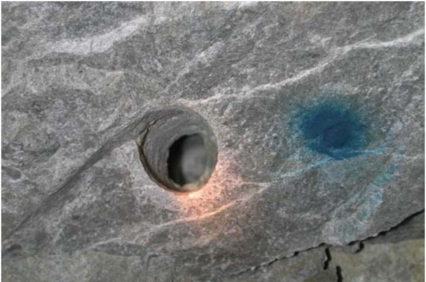
Fig. 4. Displaced borehole at site 3. Upward view on the roof; the slip-surface is sub-parallel to the roof; displacement about 15 mm.
